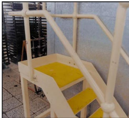
**Figure 31** Portable steps with non-slip coating applied to treads
