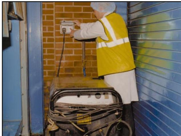
**Figure 69** Testing the RCCB on a weatherproof (IP56) socket outlet with integral RCCB protection
