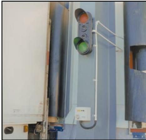
**Figure 40** Captive key and traffic-light system to prevent drive-offs at loading bay
